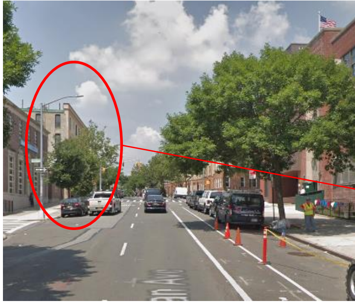
The same building can be seen on the street today in 2020.
