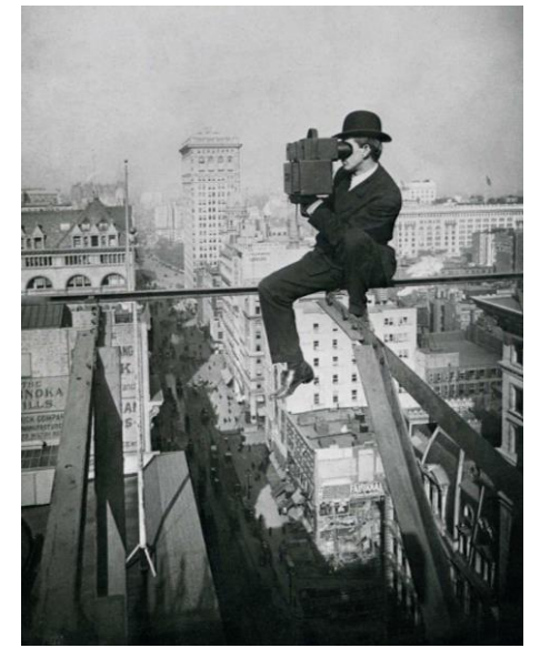
Lewis Hines in action during construction of the Empire State Building
